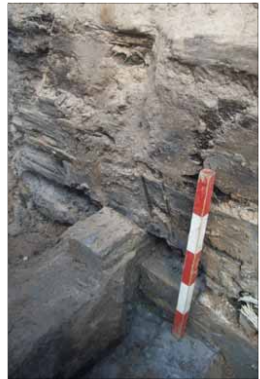
One detail of the construction of the old lock—what appears to be a tenon joint.
